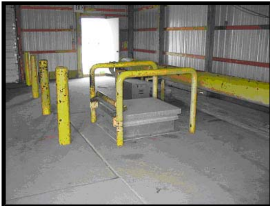
Photo 2: This lid is one of two suction ports where suction hose is dropped into the tank for drafting. The concrete floor is designed to hold the weight of the pumper.
