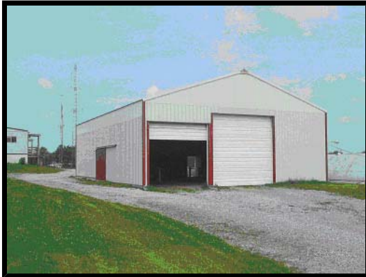
Photo 1: This metal clad structure provides protection from the elements during periods of inclement weather. Although it is not air conditioned – it could be retrofitted if needed.
