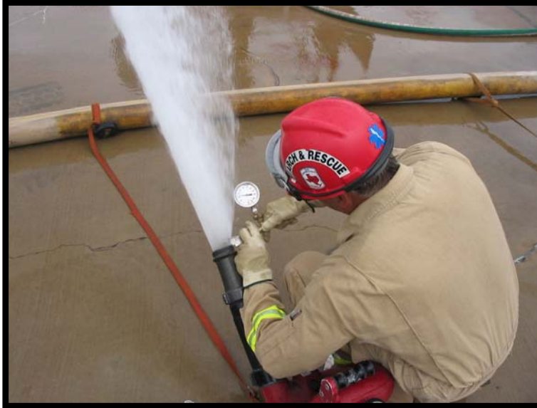
“A crew member takes a pitot reading on a 2-inch tip.”
